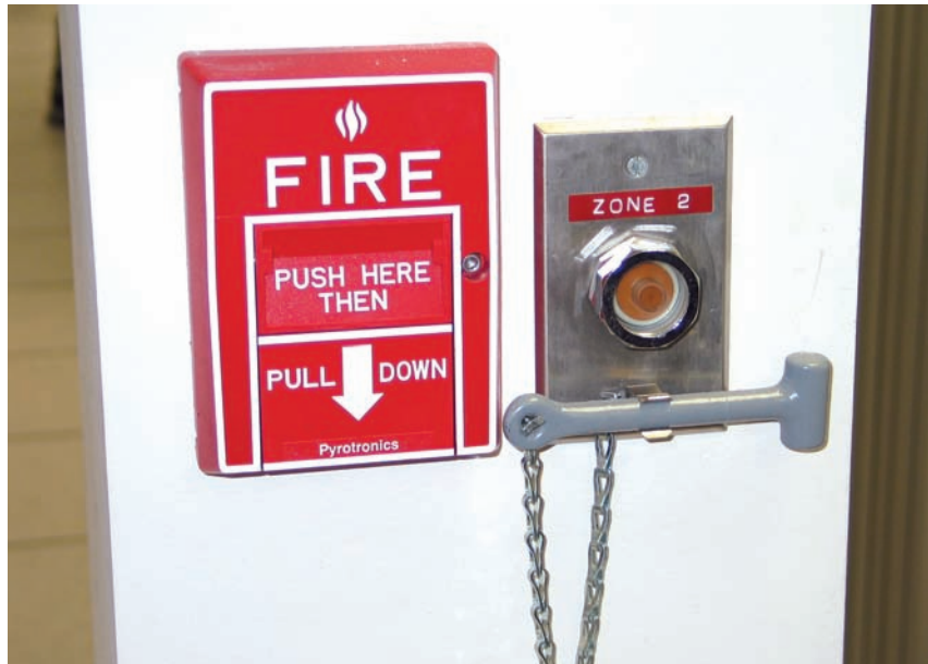
IT managers often see EPO devices as a single point of failure forced on them.
