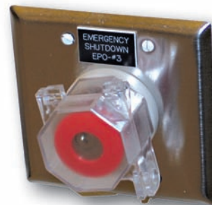
Human error is often the source of unintended shutdown; EPO devices are often the culprits.
