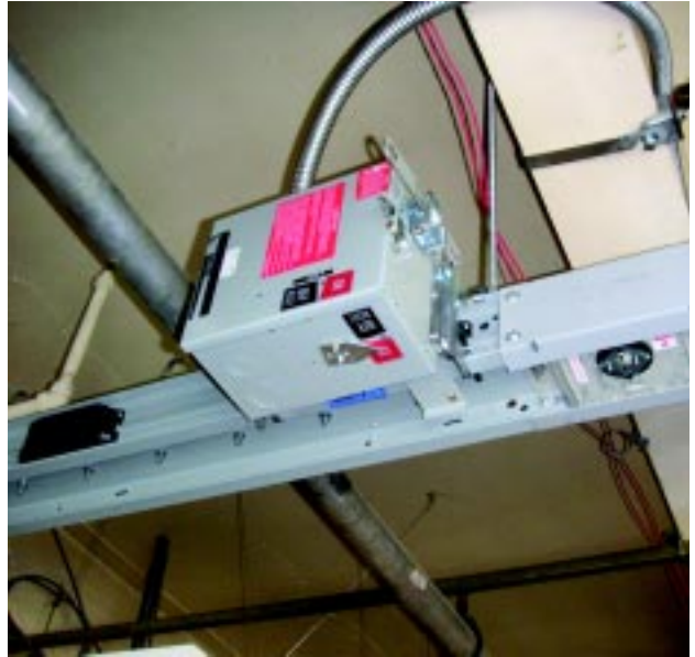
Photo 5. Circuit breaker bus plugs feature an easy-to-read position indicator, which allows maintenance personnel to quickly access system status.
