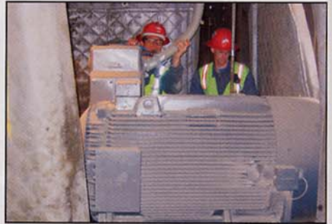
Motors play a large role in HVAC efficiency. SmithGroup, Detroit, recommends premium efficiency motors—90% efficient and higher.
