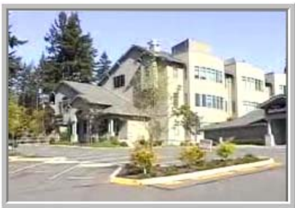
Lane Coburn & Associates, LLC - Office
